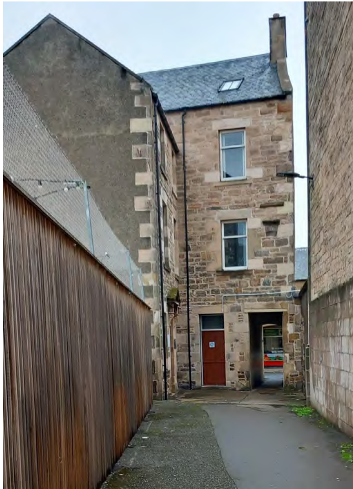
REAR VIEW OF 30-32 HIGH STREET
